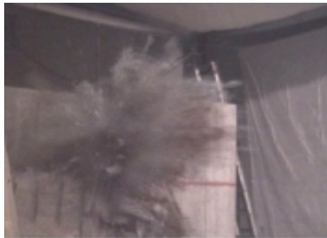
Blasting Test of Biological Shield
